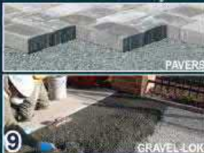
Install Surface Layer
