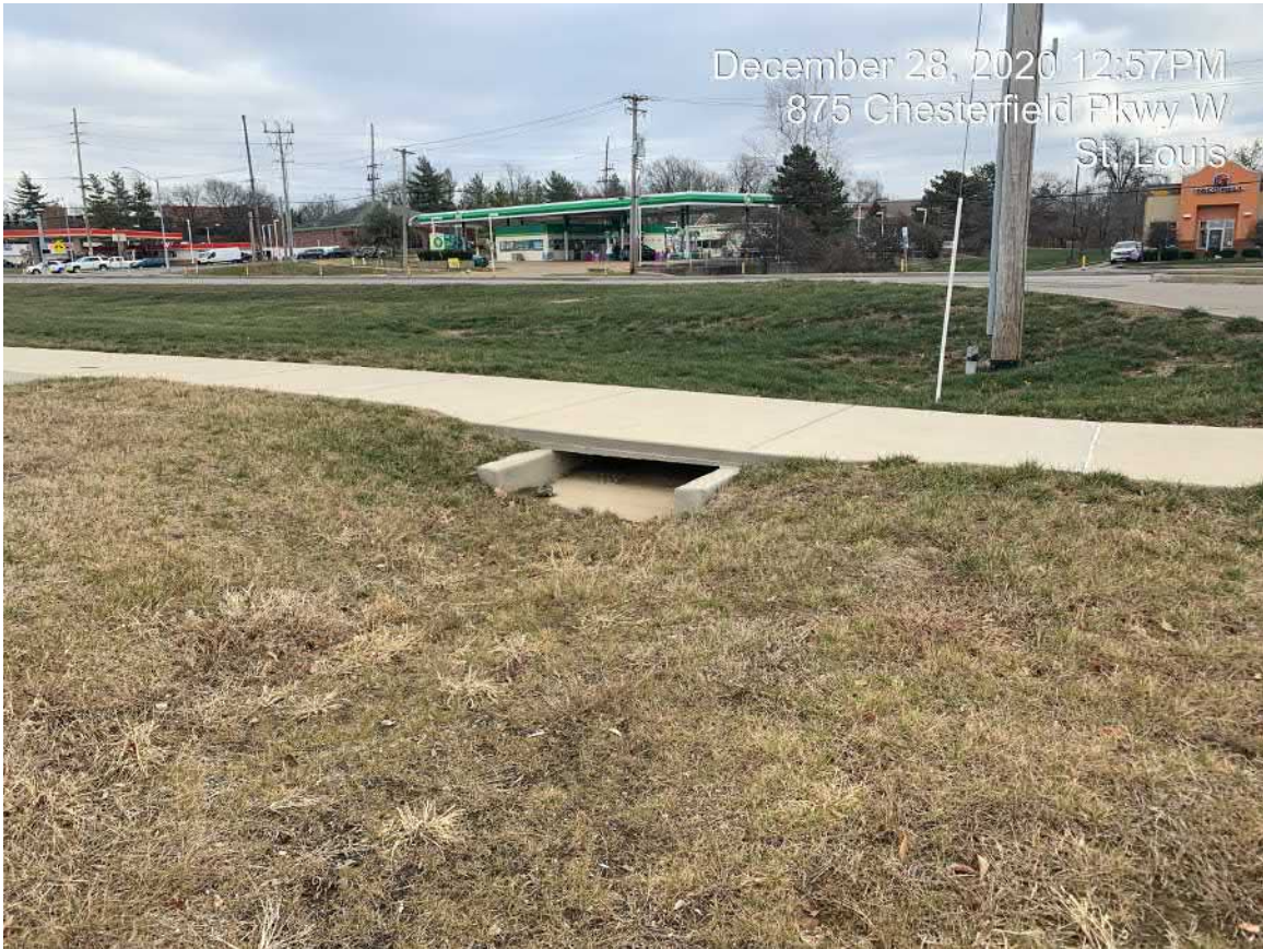
Scupper at Pfizer Office/Laboratory Along Olive Blvd.
