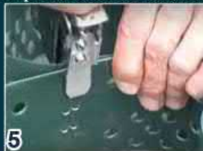
Overfill Cells & Tamp
