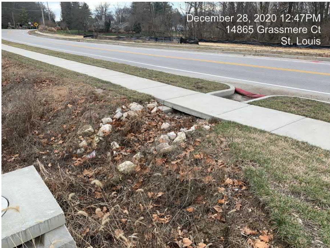
Scupper on East Side of Schoettler Road south of the Schoettler Road Bridge.
