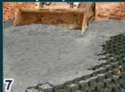
Completely Fill Cells
