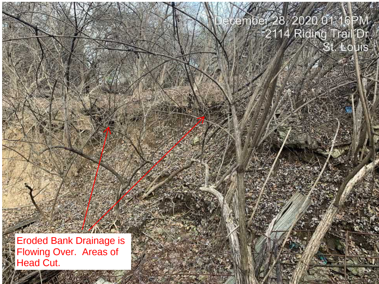
Unstable Bank of Existing Drainage Way. Looking From Flow Line of Drainage Way.
