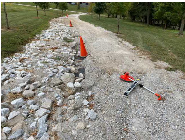
Figure 4: West end of north leg of South Trail loop. Geofabric exposed after continued erosion.
