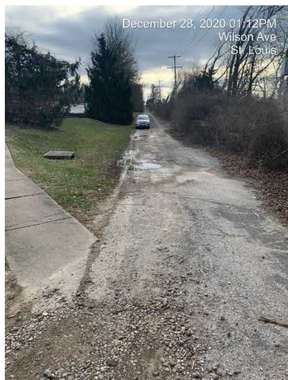
Existing Access Drive to 2153 Wilson Ave.
