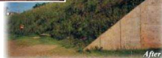
Roadway lane expansion project with reinforced soil slope up to 30 feet tall, spray seeded with native material.
