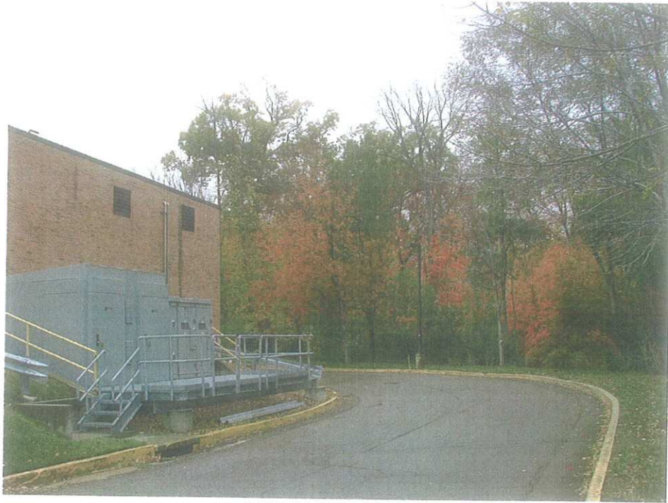
VIEW LOOKING NORTH FROM ACCESS DRIVE
