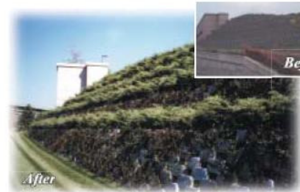
Parking lot expansion vegetated with Euonymus vines.
