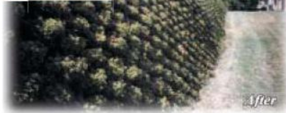
Apartment community tie wall replacement
