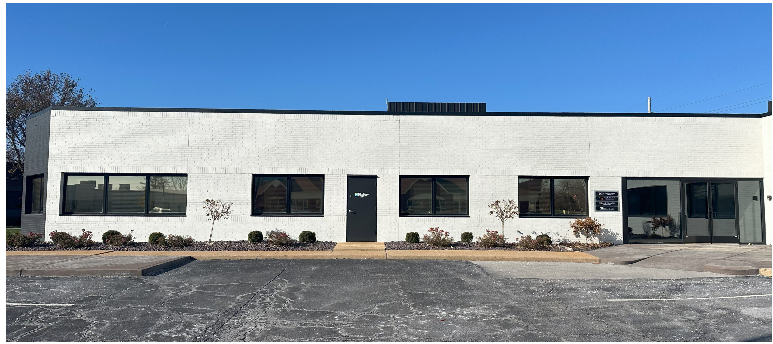
6 | Partial East Exterior Building Elevation - Near Entry Door A101 | Not To Scale
