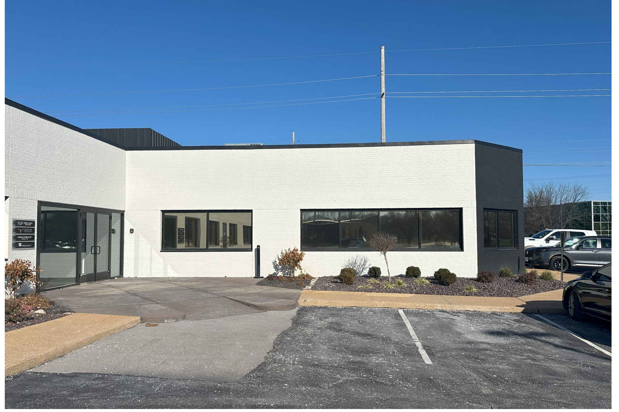
1 | Partial South Exterior Building Elevation - Near Entry Door A101 | Not To Scale
