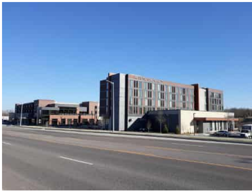
AC HOTEL CHESTERFIELD - NORTH OF SITE
