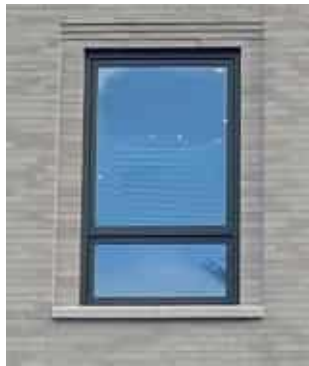
ALUMINUM CLAD WINDOWS (PUNCHED WINDOWS) EXAMPLE PHOTO
