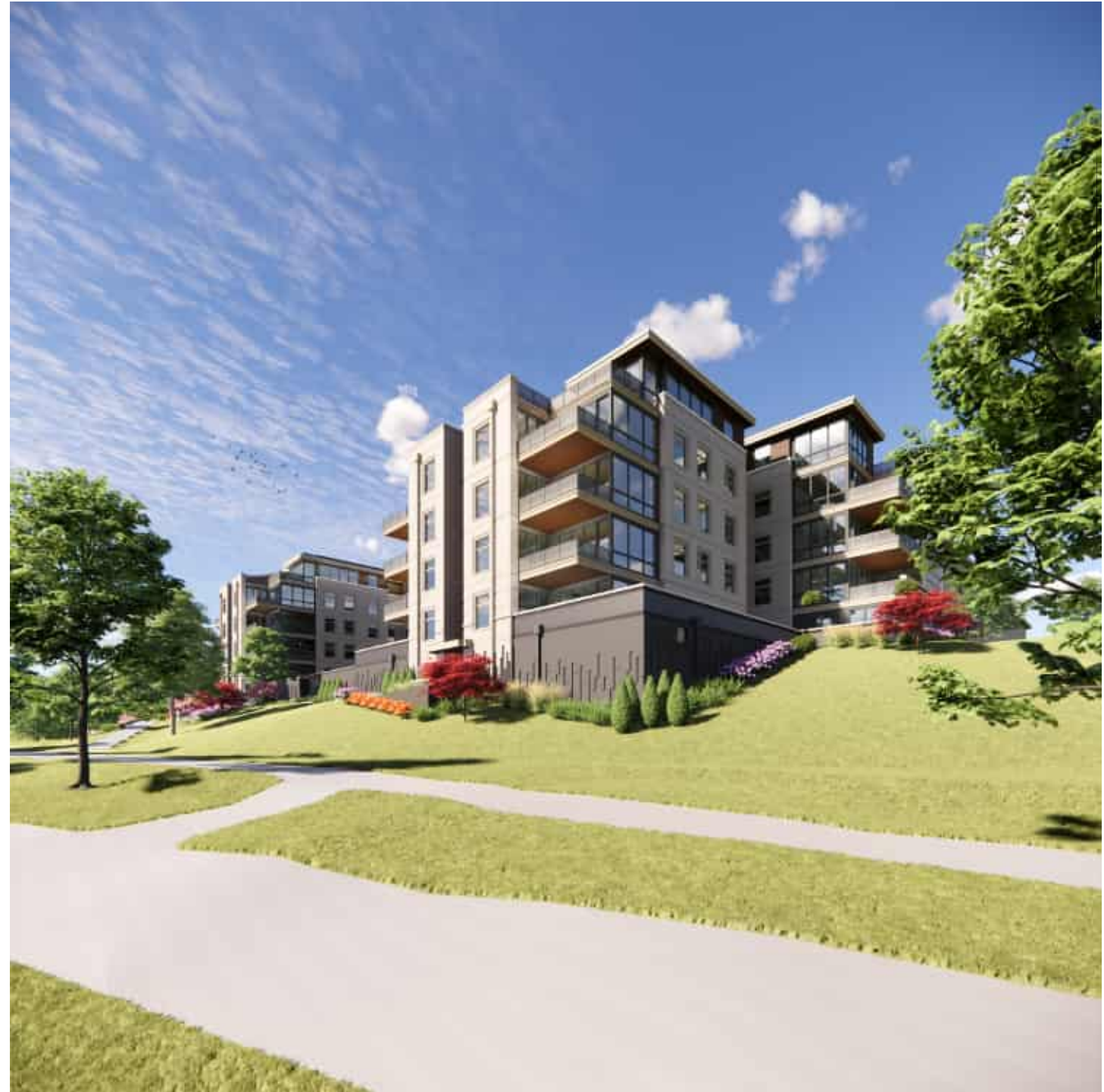
CORNER VIEW FROM LAKE SIDE
