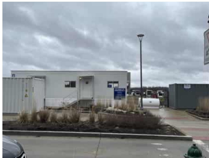
VIEW LOOKING SOUTH AT PROJECT SITE
