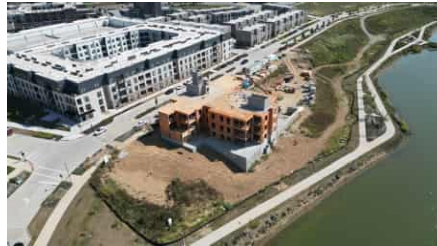
AERIAL VIEW LOOKING NORTHEAST OF PROJECT SITE
