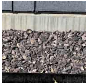
GRAVEL MAINTENANCE STRIP (SEE LANDSCAPE) 3/4" - 1" CLEAN ANGULAR TRAP ROCK 5" X 1/4" STAKED STEEL EDGING, BLACK POWDERCOAT
