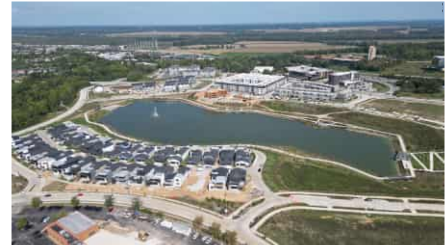
AERIAL VIEW LOOKING NORTH ACROSS LAKE OF PROJECT SITE
