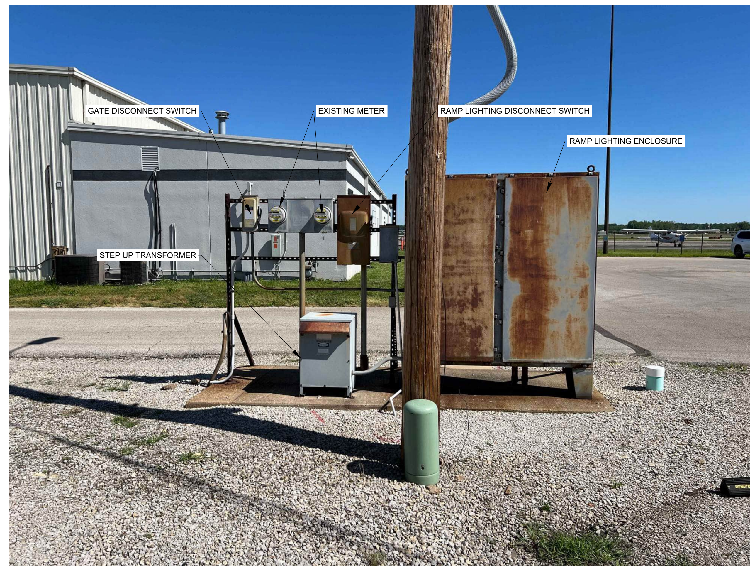
1 EXISTING POWERFRAME TO BE RELOCATED N.T.S.
