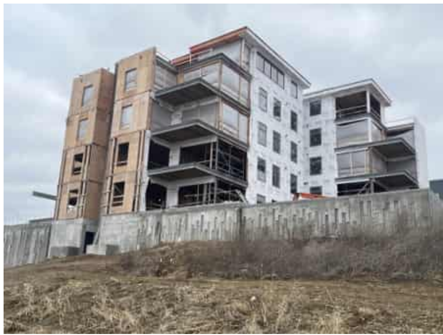
VIEW LOOKING NORTH AT ADJACENT BUILDING TP PROJECT SITE
