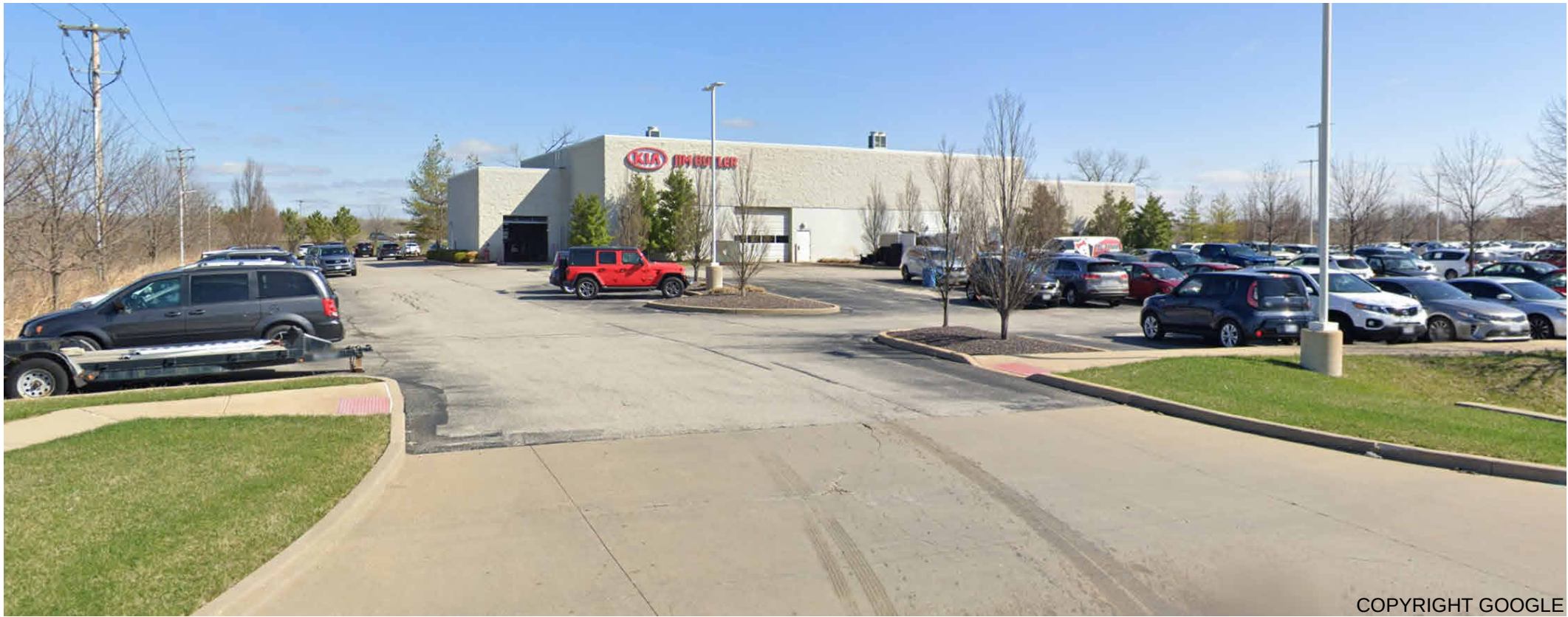
EXISTING BUILDING (NORTH OF SITE)
