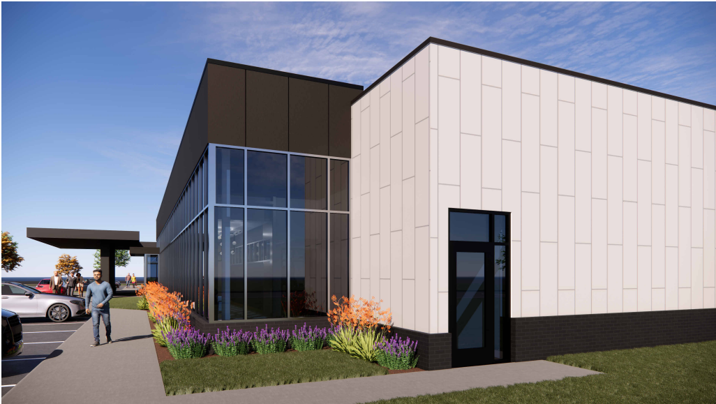
SOUTHWEST CORNER VIEW
