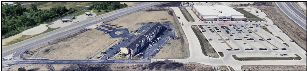
Figure 2: Existing Site, Google Earth 2023
