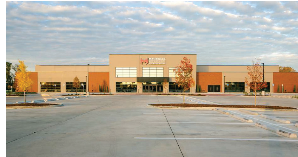
VIEW OF EXISTING BUILDING FROM PARKING LOT
