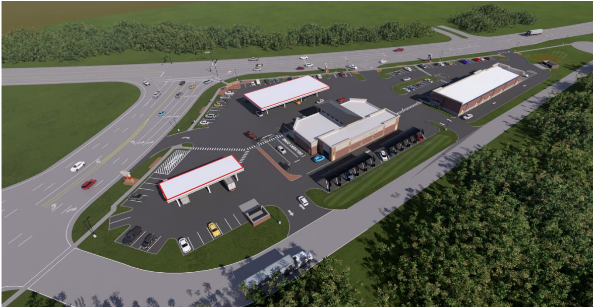
Aerial view from Old Olive Street Road
