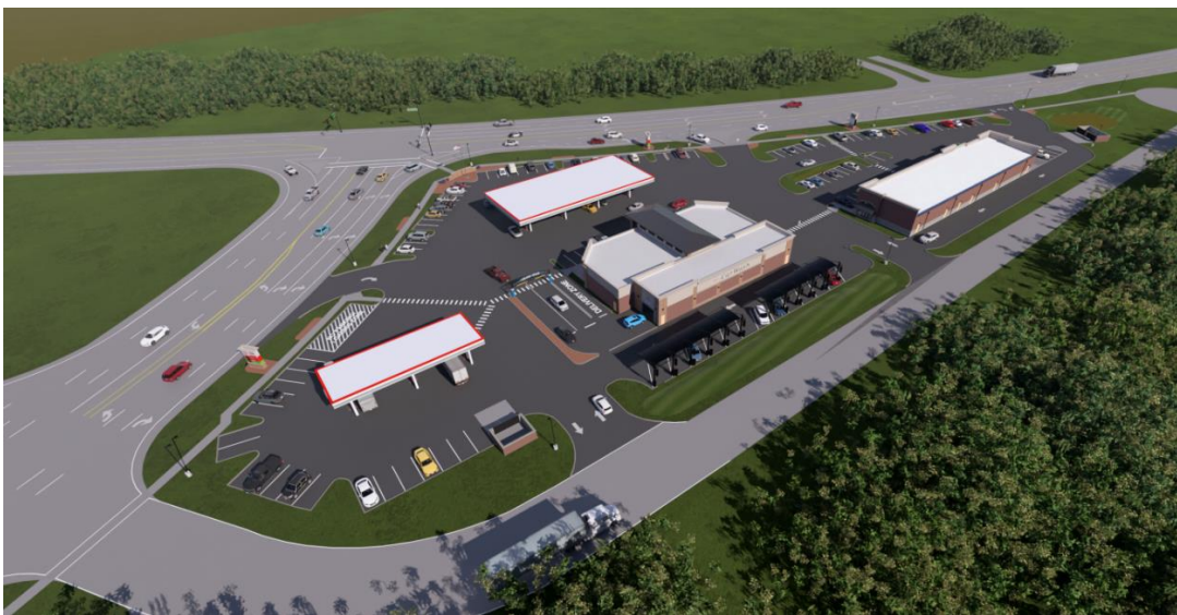
Aerial view from Old Olive Street Road
