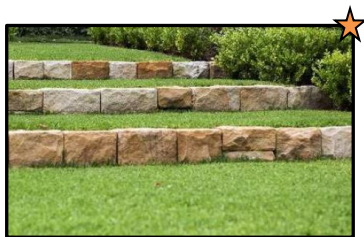
Figure 13: Limestone mill block seating and retaining wall
