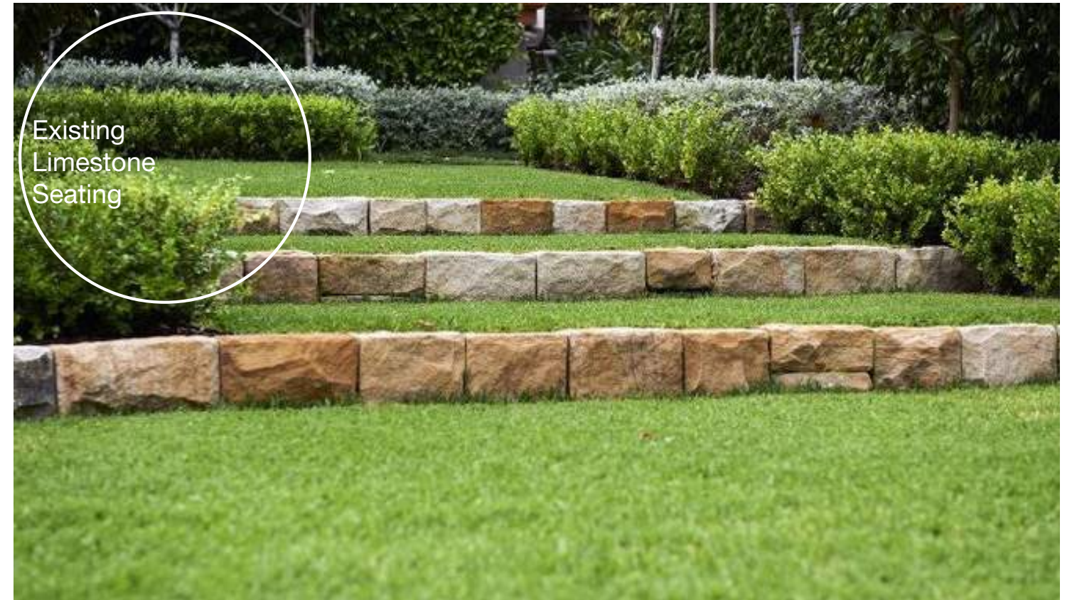
LIMESTONE MILLBLOCK SEATING AND RETAINING WALLS
