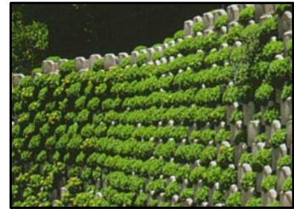
Figure 18: Alperstein retaining wall
