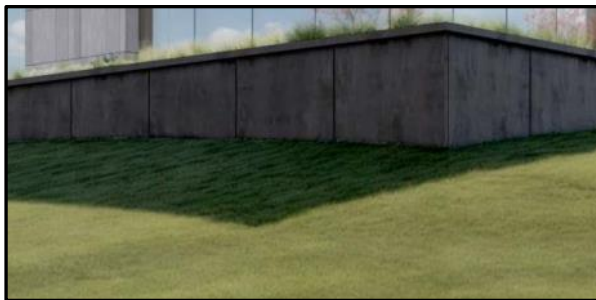
Figure 17: Concrete retaining wall with formliner
