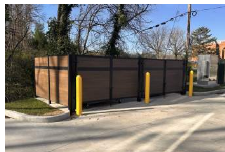
SIDE PHOTO TRASH ENCLOSURE
