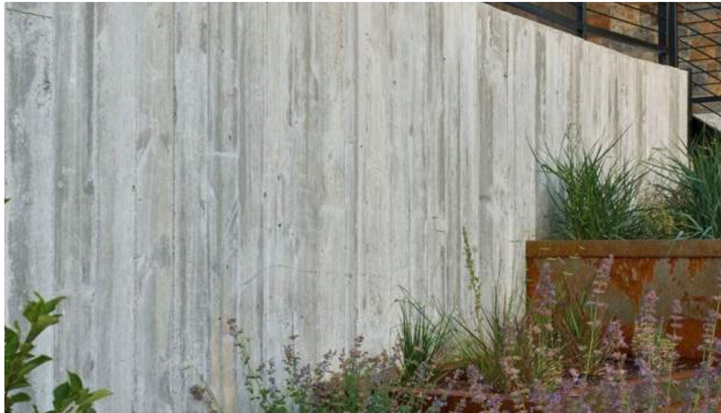
CAST IN PLACE CONCRETE RETAINING WALL WITH FORMLINER
