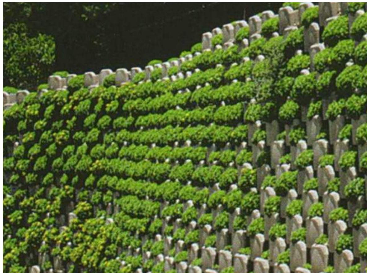
ALPENSTEIN RETAINING WALL
