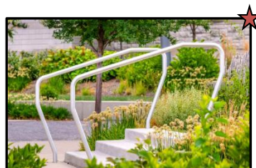
Figure 14: Concrete stair with railing
