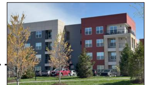
PARQ AT CHESTERFIELD APARTMENTS
