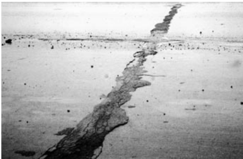
► ► Cracks parallel to joint. Dark color next to transverse joint likely indicates D-cracking and additional deterioration. Full depth repair required.
