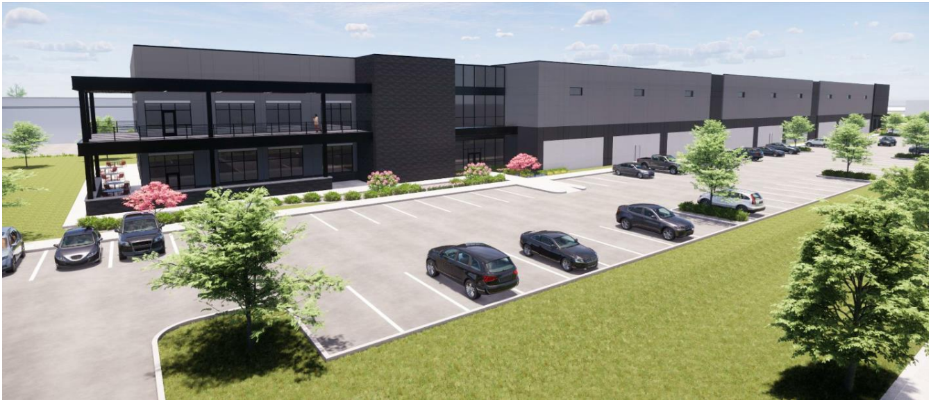
Aerial view from Wings Corporate Drive.
