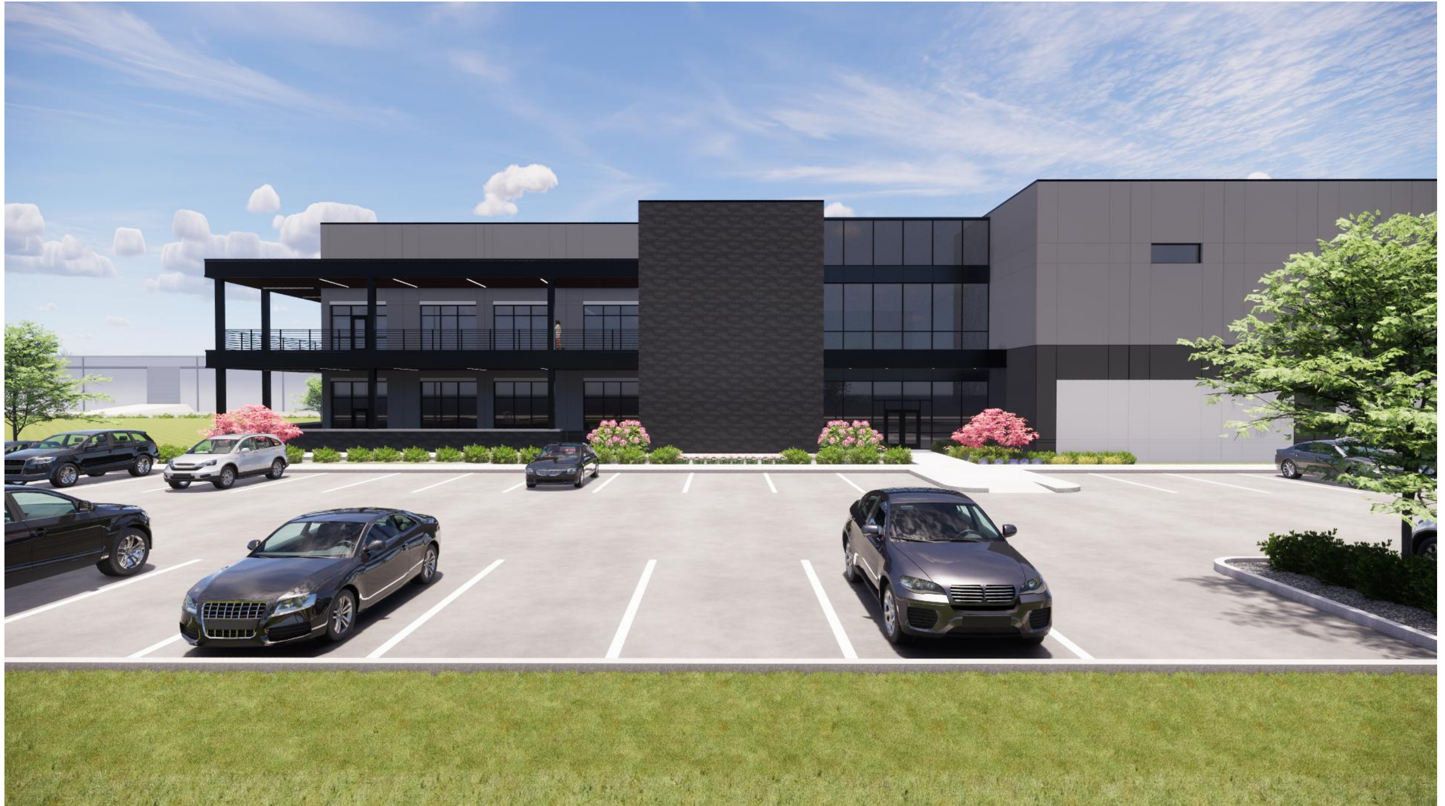
NORTHEAST SIDE SHOWING STONE CLAD WALL AND MAIN ENTRY
