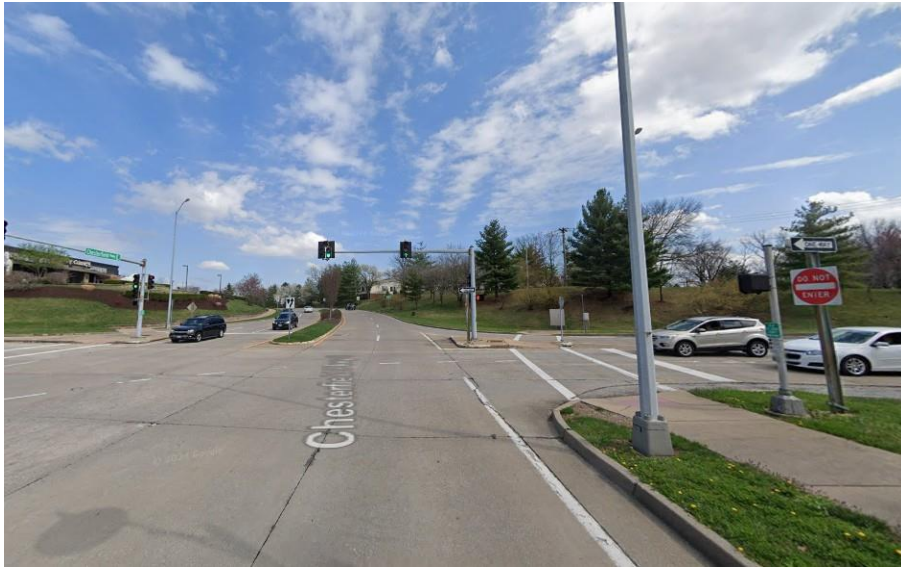
(Chesterfield Parkway at Clarkson Rd off-ramp)
