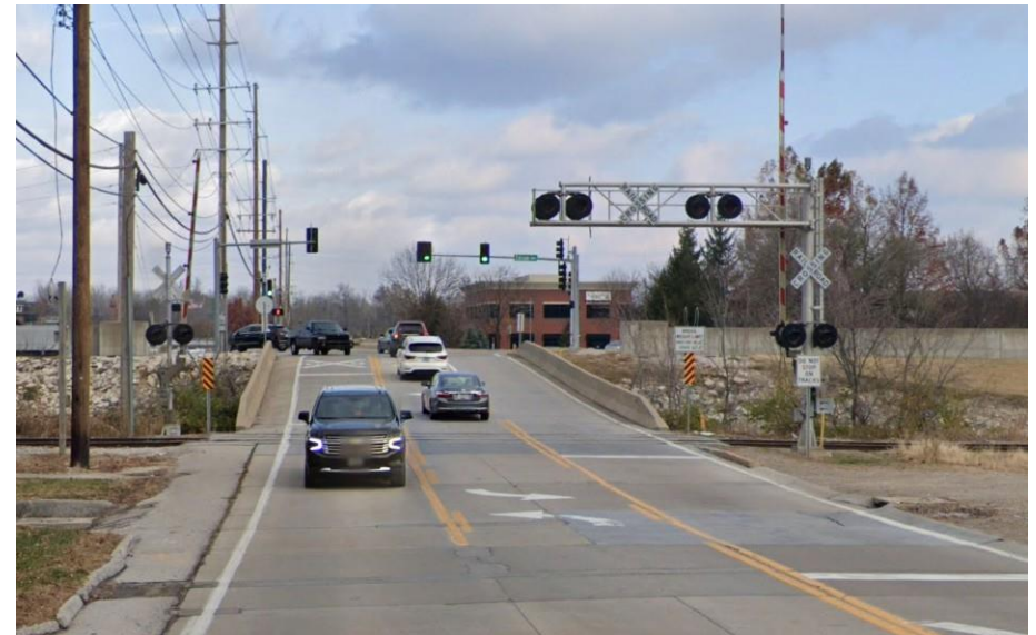
(Baxter Road at Bonhomme Creek Bridge)
