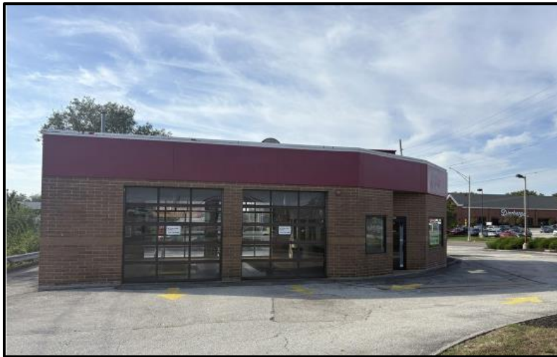
Figure 6: Existing view of building from Olive Blvd.
