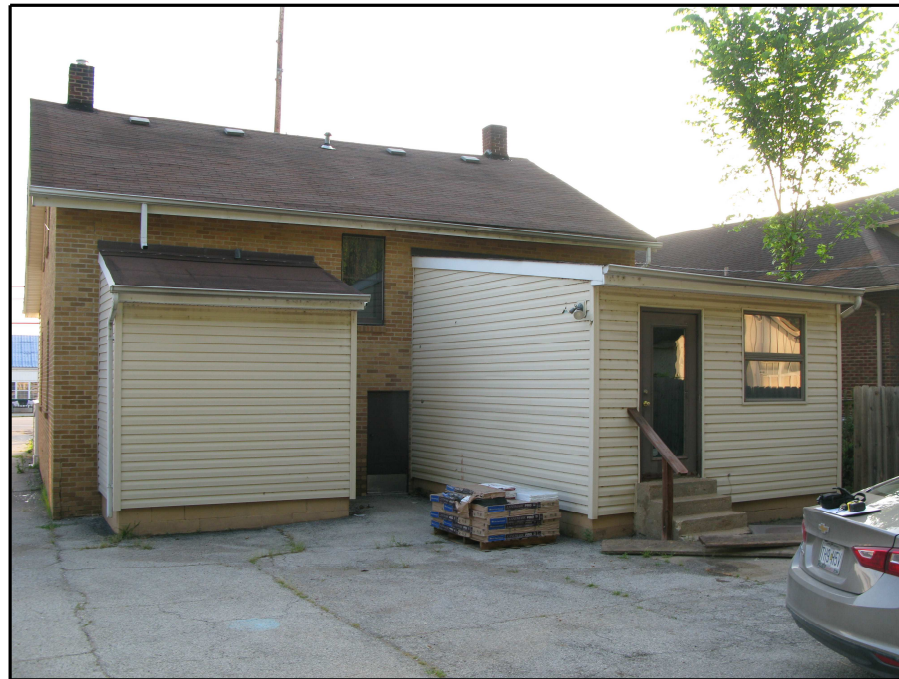
EXISTING BUILDING VIEW FROM SOUTHWEST
