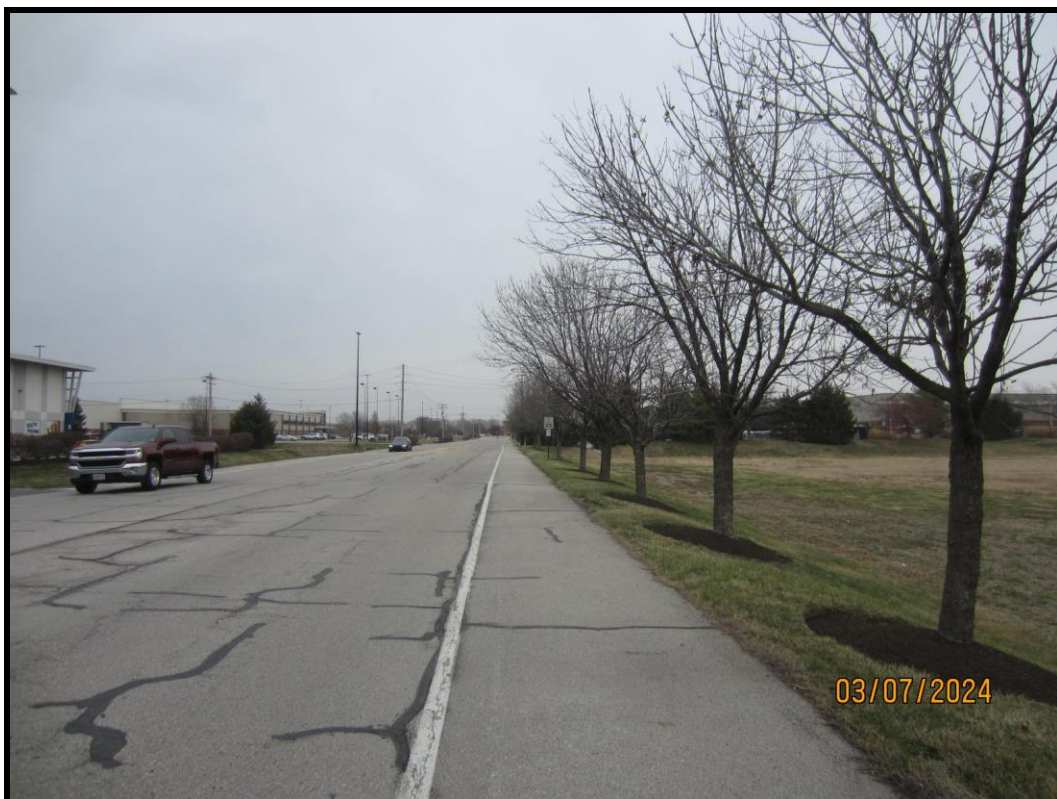
Subject Property – Looking North along RHL Drive
