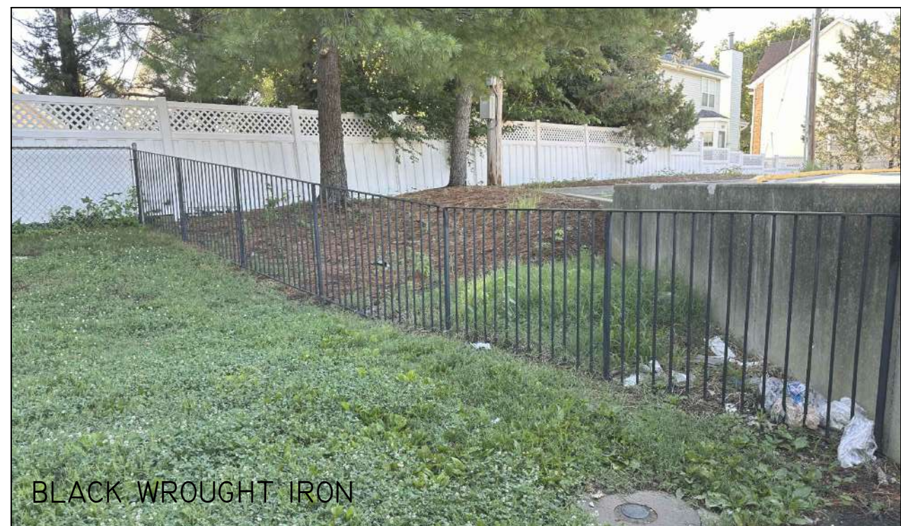
12 PHOTO OF EXISTING FENCE, EAST A.II
