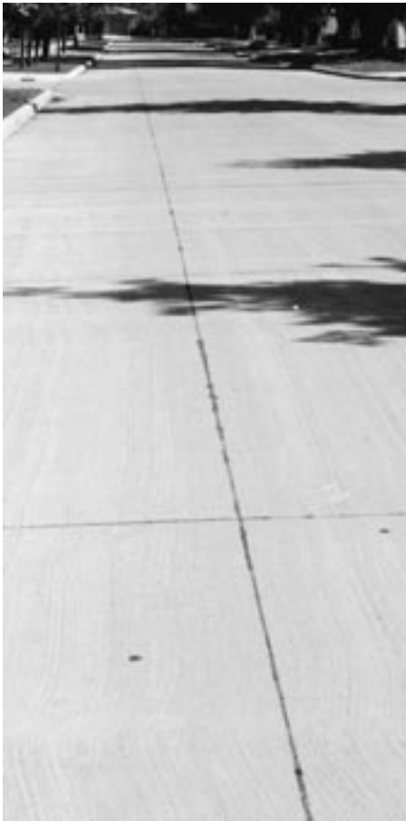
◀ New, well-sealed longitudinal joint.
