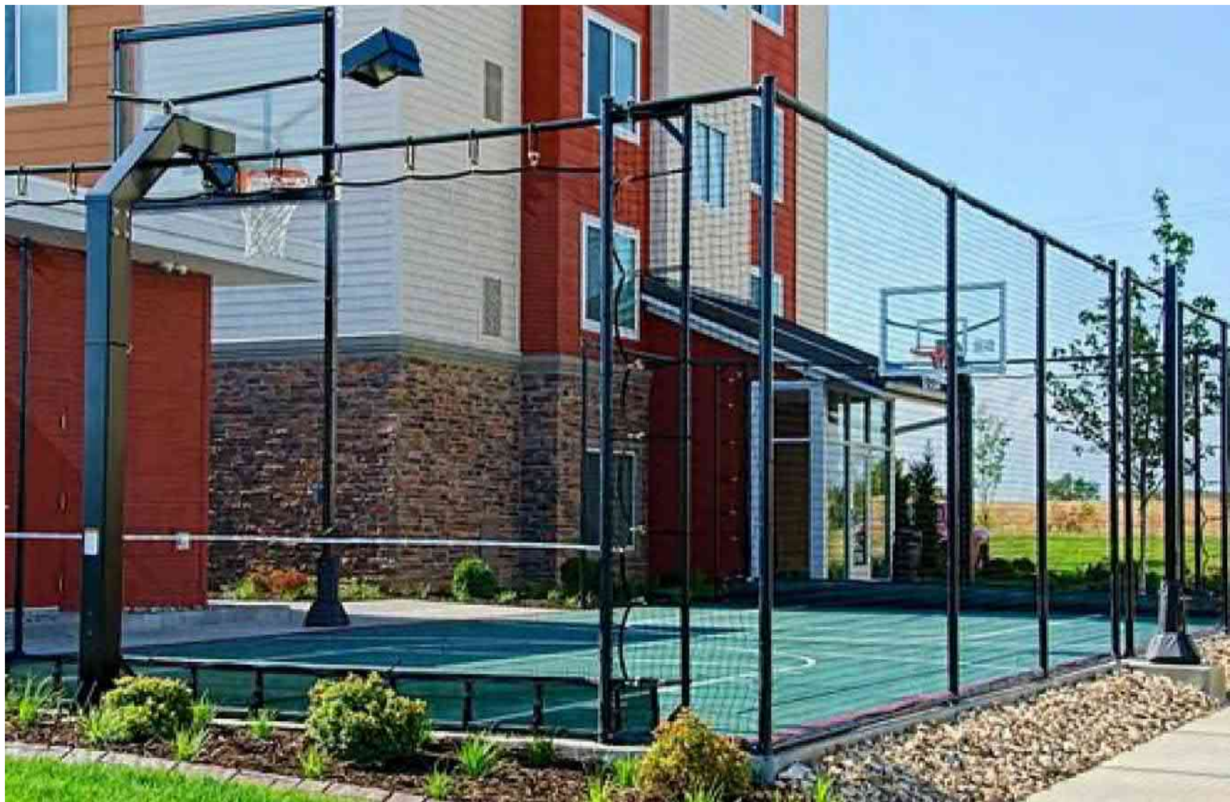
SPORT COURT FENCE DETAIL (N.T.S.) NOTE: SPORT COURT MATERIALS: 1. POWDER COATED STEEL POLES 2. 10' UV-PROTECTED MESH NET
