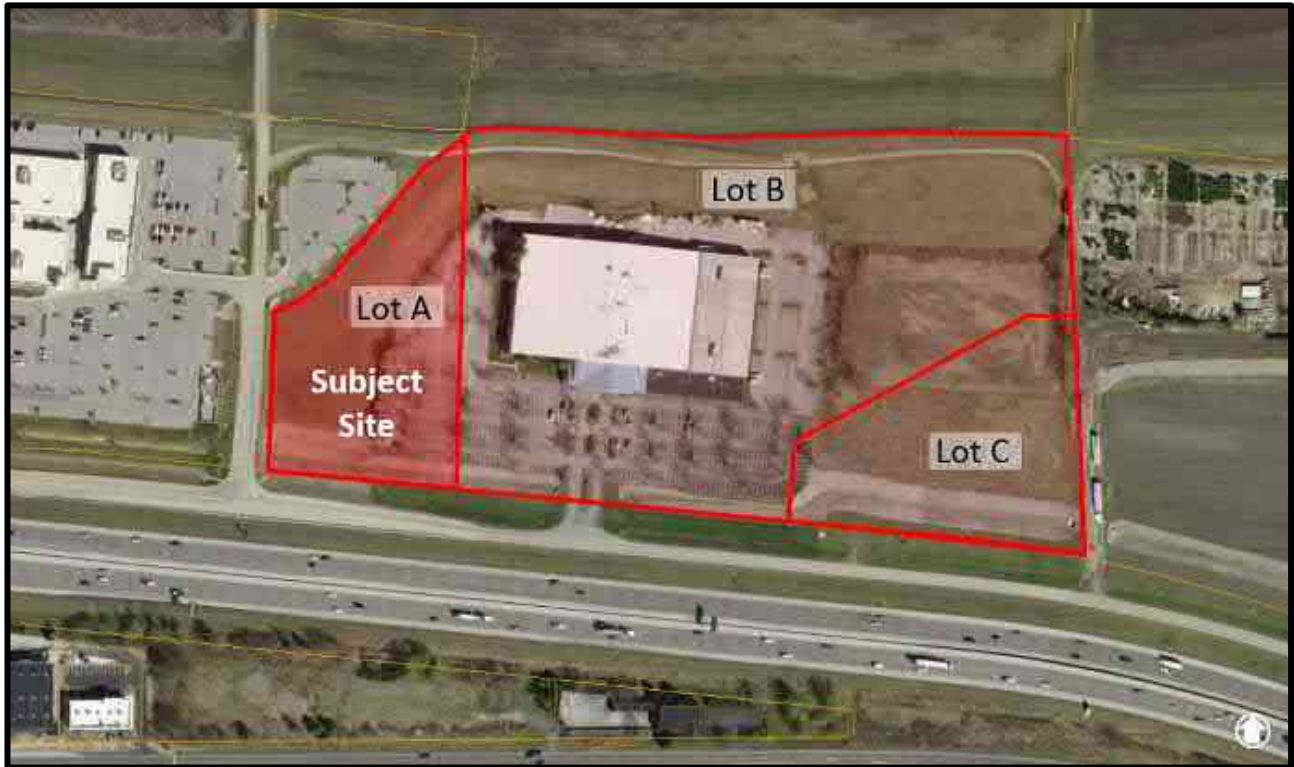
Figure 1: Aerial Site Photo
