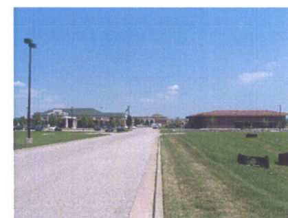
VIEW FROM LOCATION "B" LOOKING EAST
