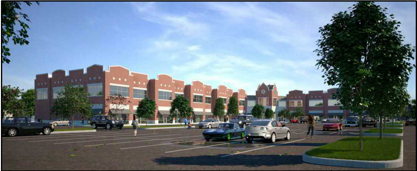
Figure 9: Retail/Office Buildings (North)
