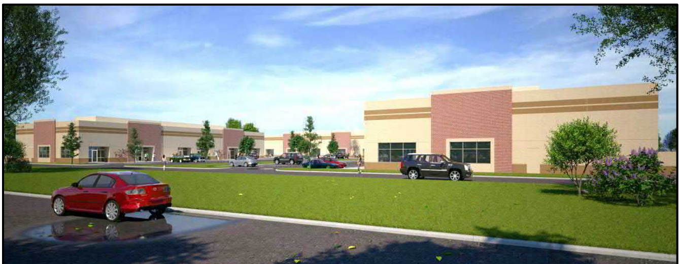
Figure 8: Warehouse/Office Buildings (North)
