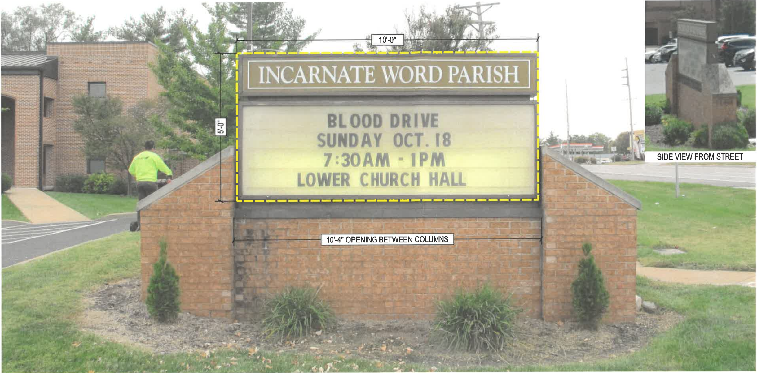
EXISTING DOUBLE-FACE INTERNALLY-ILLUMINATED MONUMENT SIGN - REMOVE ID. & CHANGER CABINET. / LEAVE BRICK BASE & METAL FLASHING (REPAINT FLASHING ON-SITE). SCALE: 1/2" = 1'
