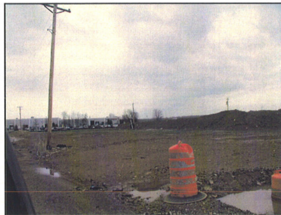
View Looking north from Lot 3
