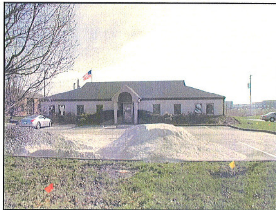
Existing building on site
