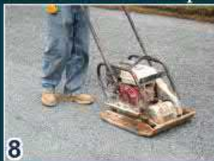
Overfill Cells & Tamp
