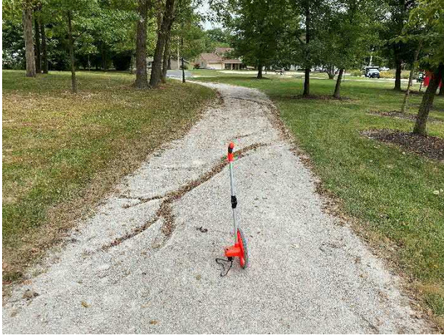
Figure 11 – Northeast corner of the North Trail, facing east, erosion occurring from stormwater draining from the north (left in photo).
