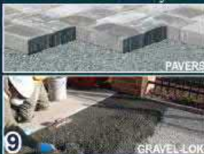
Install Surface Layer
