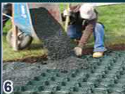
Install Surface Layer
