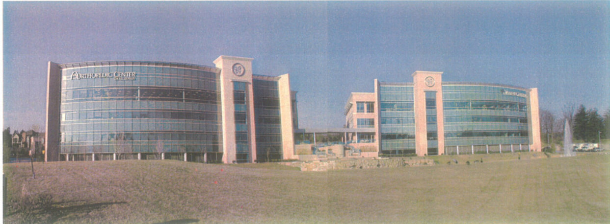
Existing buildings on the site.
